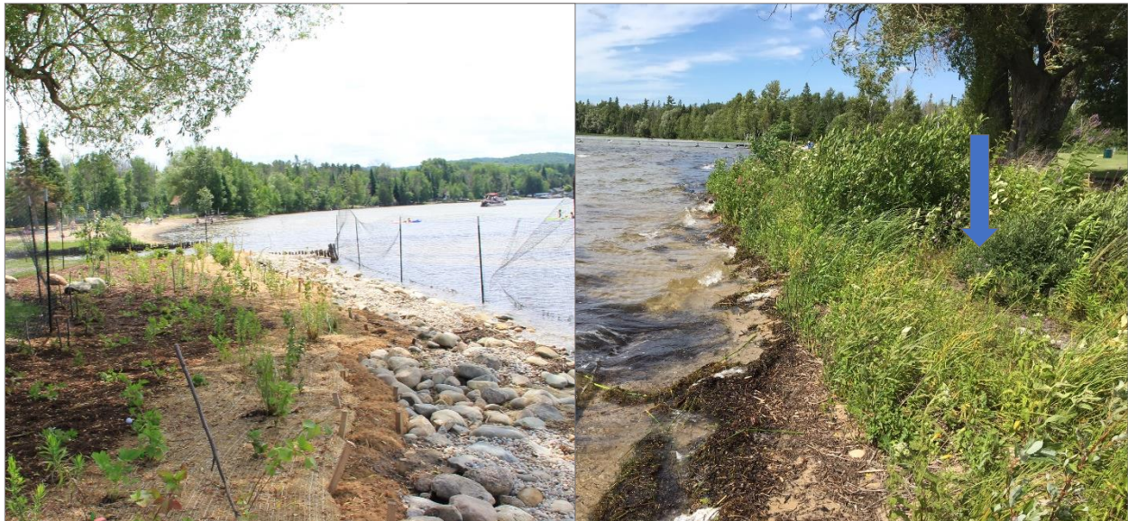
Bioengineering demonstration site at Camp Pet-o-se-ga shortly after installation in 2014 (left) and six years later (right). The blue arrow shows the location of the coir log, now covered with thriving native plants.
